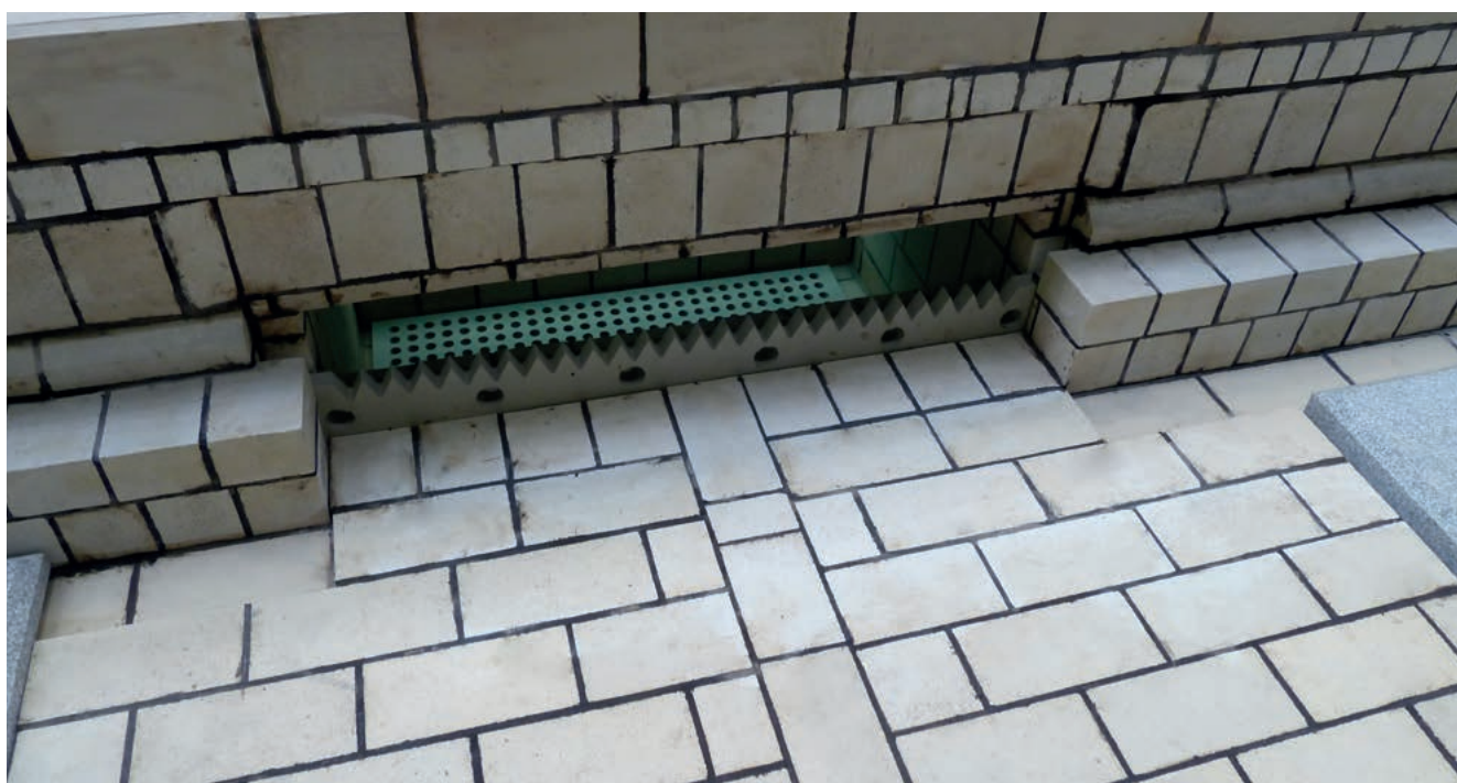
Brick lining with CHEMOKITT FU 1310
